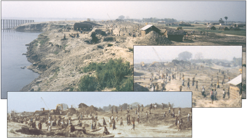
Figure 1.3: People in action to shift the flood-defence embankment near Kamarjani. On the left hand side one of the permeable groynes (consisting of a set of piles) that was tested as part of the Bank Protection and River Training Pilot Project (FAP21/22).
